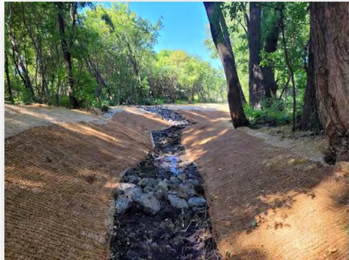
(Above) Placing veins of rip rap (larger diameter rock) along the channel helps disperse stream flow energy, keeping channel sediment in place.
