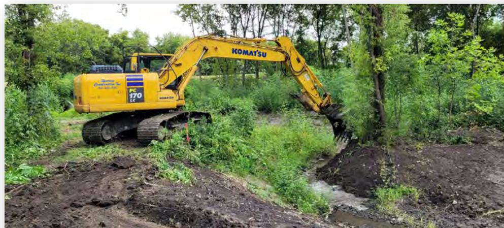
(Left) Reshaping bank slopes takes place prior to spreading of native seed and stabilizing using erosion control blanket along the south channel of the restoration. All up-slope areas that equipment used to access bank slopes were seeded with a native ground cover and stabilized using straw mulch.
