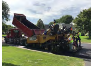
Installation of new asphalt surface
