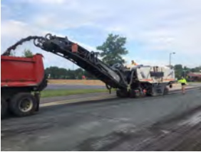
Removal of existing street surface by milling
